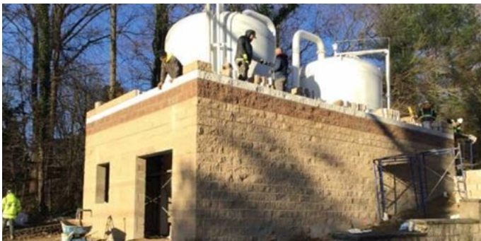
One of three additional PFAS Treatment Building Under Construction.
